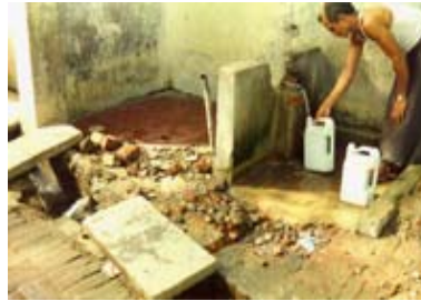
Unhygienic Community Water Supply
