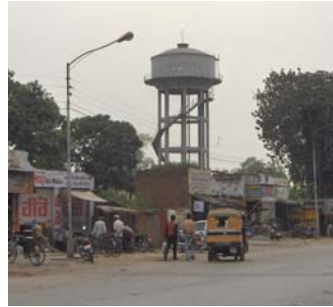
Over Head water Reservoir
