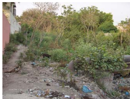
Drain chocked with solid waste near Hindustani Basti
