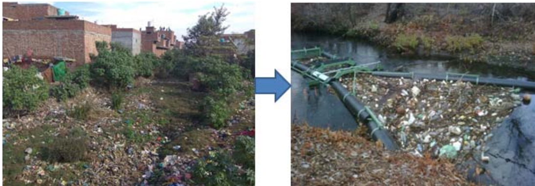
Photograph 2-2: Current and proposed condition of open Ganda Nallah at Bengali Basti
