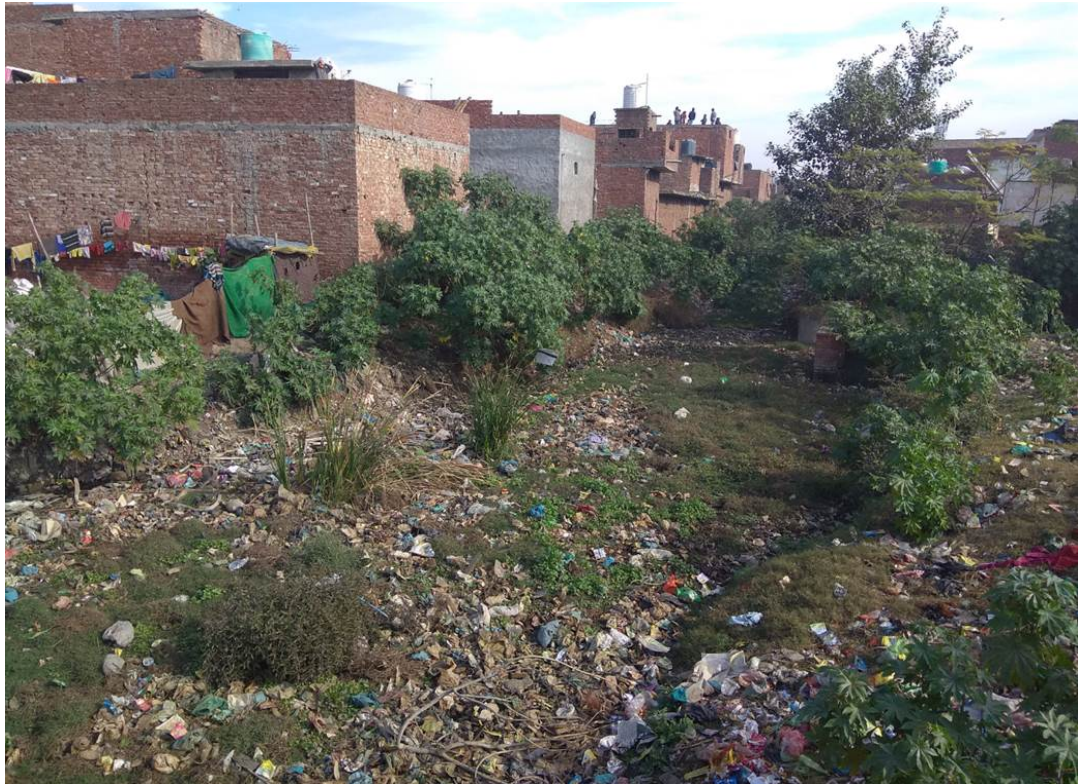
Photograph 2-1: Heavily silted open Ganda Nallah at Bengali Basti
