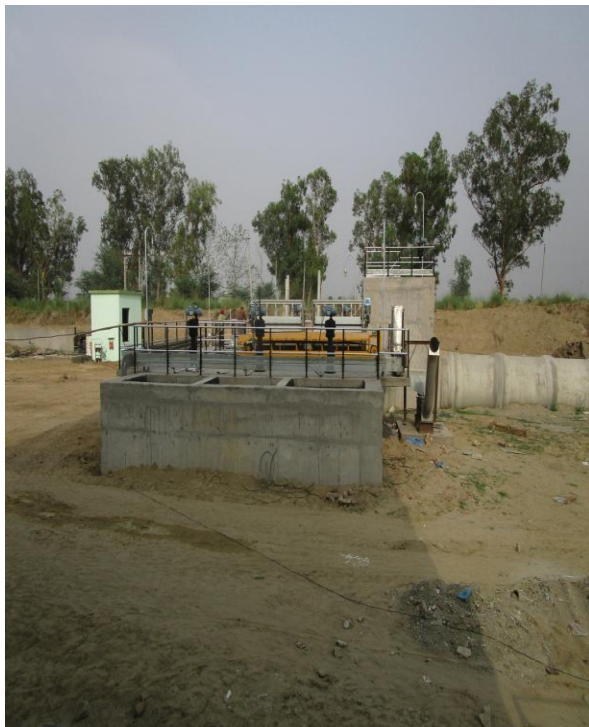
MAIN PUMPING STATION INLET:-
