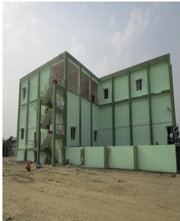
MAIN PUMPING STATION:-
